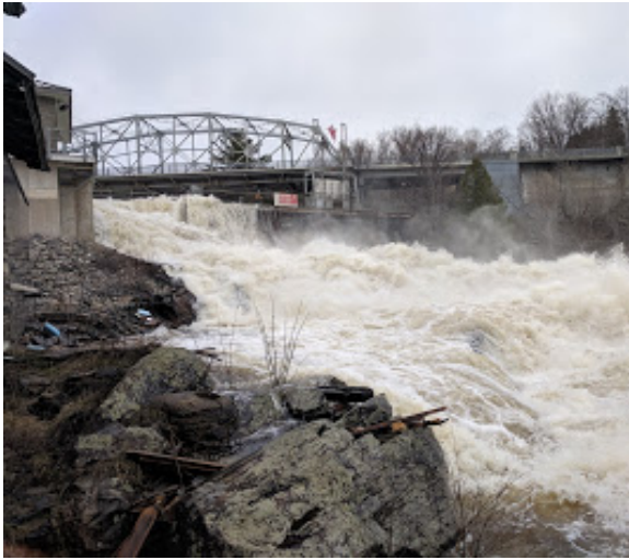
High-volume of flood water flow over the dam near Ecclestone Drive in Bracebridge (April 29, 2019, pictured by Jack Rozdilsky)
